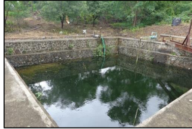
Rain water Pond No. 2
