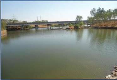
Rain water Pond No. 1
